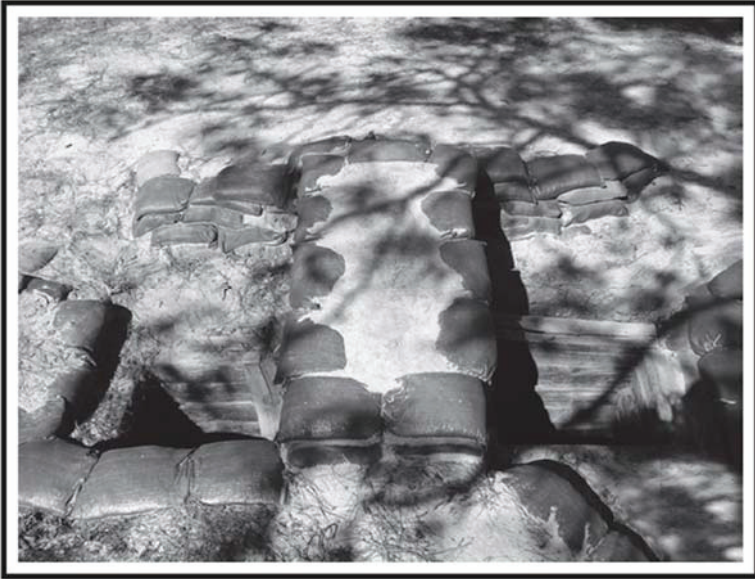
071-COM-4408-8. Machine gun fighting position with OHC.
