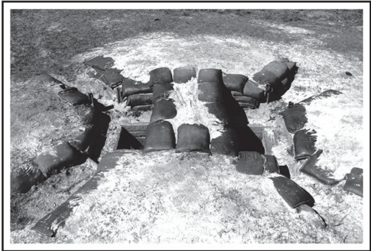
Figure 071-COM-4408-2. Two-man fighting position with OHC.
